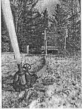
RIPTON FIRE RESCUE on Oct. 18 performs a flow test of the recently installed dry hydrant on private property off Fire Brook Road. A dry hydrant is not connected to a water source but instead draws water from a pond or stream for firefighters to use in fighting fires in the neighborhood. Below, water flows from the private dry hydrant sitting out of the ground on the left, through the 6-inch pumper tank and out of a fire hose. The newly installed dry hydrant passed the test. Photos courtesy of Chris Pike.
