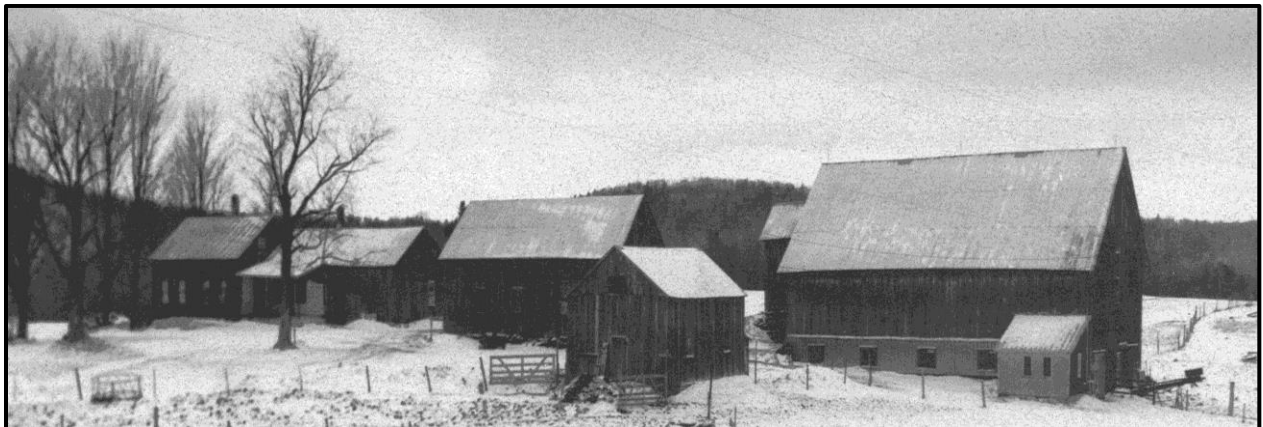
The Malone Farm in East Bakersfield includes an 1850 house on the left and a high bank dairy built in 1890 on the right. Horses pulled hay wagons piled high with loose hay up the ramp or wharf. Hay was packed into the sides of the loft and dropped down to the dairy cows in the ground floor stable below. Credit: Bakersfield Historical Society.
